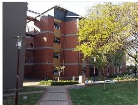
Student residence at Onderstepoort, University of Pretoria (Corobrik)
