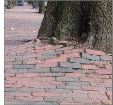
Pavements constructed with segmental pavers are much easier to repair than poured concrete, resulting in simpler and less costly maintenance.
