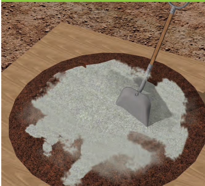
8.14 - Spread the cement over the mixture.
