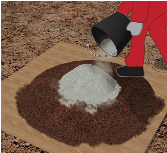
8.13 - The bucket of cement is emptied on top of the six buckets of sand and the bucket of lime.
