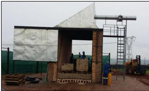
Figure 4: On-going model kiln packing process
