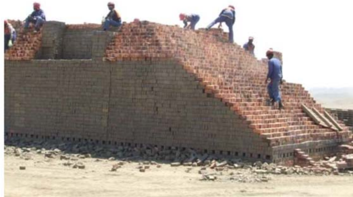
Figure 6: Example of a clamp kiln in preparation (Rice, 2012).
