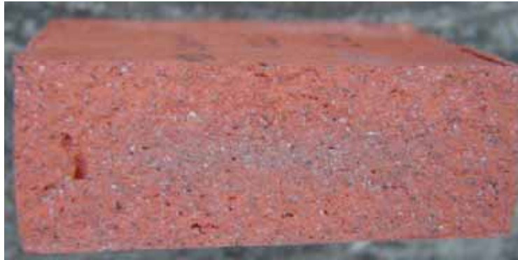
Broken brick face
