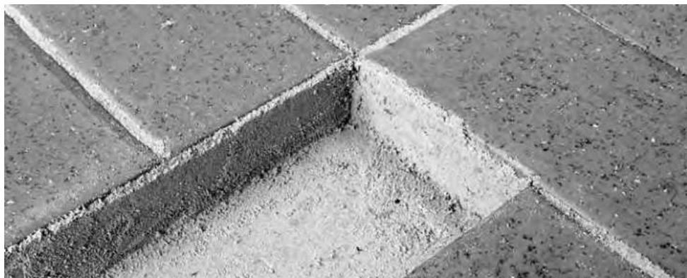
Figure 4 Well-filled sand joint
