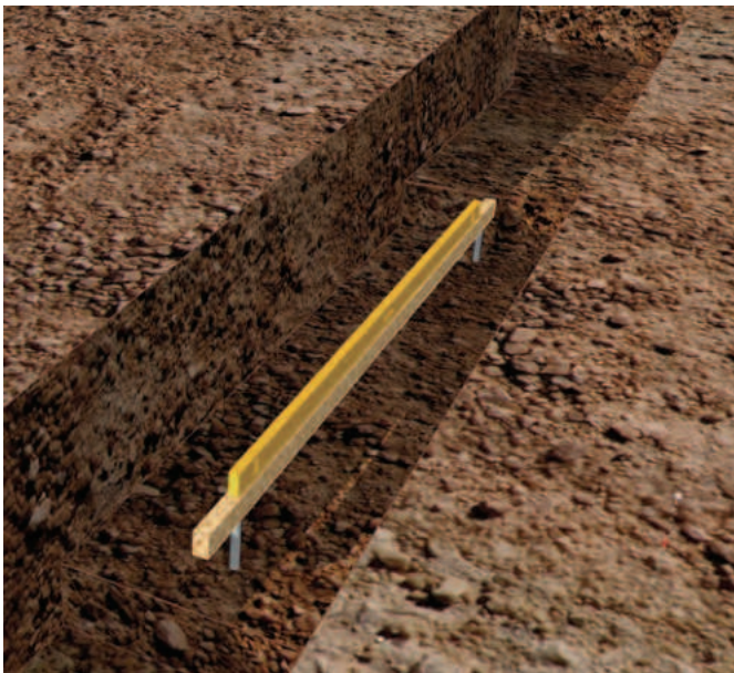
5.14 - Level pegs are then driven into the bottom of the trench starting at the lowest point and allowing the first peg to protrude 225 mm above the bottom of the trench. Use a 2 m straight-edge and drive in the next peg slightly less than the length of the straight-edge away from the first peg. The top of the second peg is levelled with the top of the first, using the straight-edge and spirit level. This process is continued along the trench until the last peg to be driven in level protrudes less than 150 mm above the bottom of the trench. At this point another peg is driven in next to the last peg, but with its top about 90 mm higher. At this point the foundation will later be stepped.
