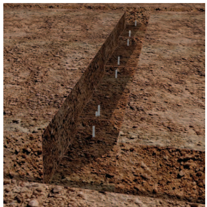
5.16 Level pegs in position.
