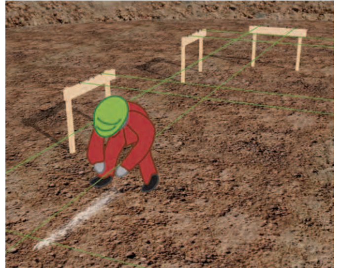
5.12 -The foundation measurements can also be transferred down by pouring lime or sand on the ground below foundation lines.
