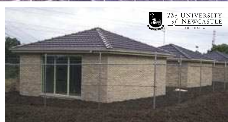
Figure 3 Test building modules at The University of Newcastle.
