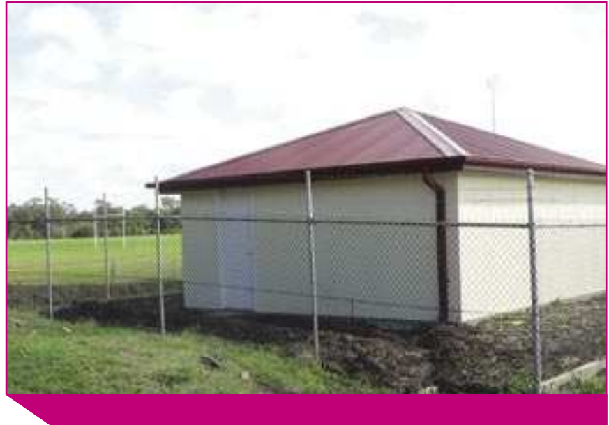
Figure 14 Lightweight test building module at The University of Newcastle
