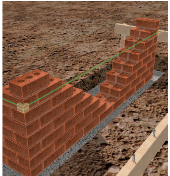
11.15 - Filling in the brickwork between corners, a builder's line and line-blocks or line-pins are used to ensure that each course is laid straight.
