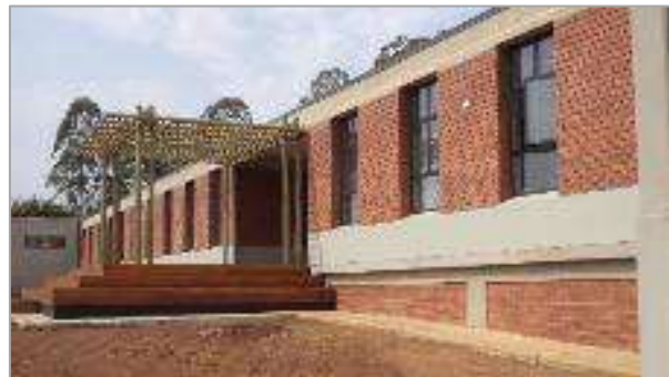
5-star rated Green Building - KZN Department of Public Works' Sisonke District Office in Ixopo (Photograph courtesy of Corobrik)
