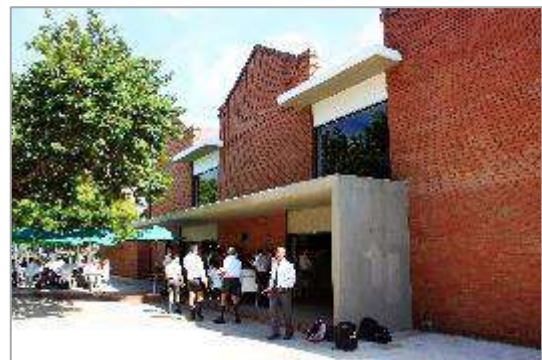
Afrikaans Seuns Hoerskool in Pretoria matched the red brick from the original 1929 building when they extended their learning centre in 2013, to ensure a uniform appearance. Photograph courtesy of Corobrik.
