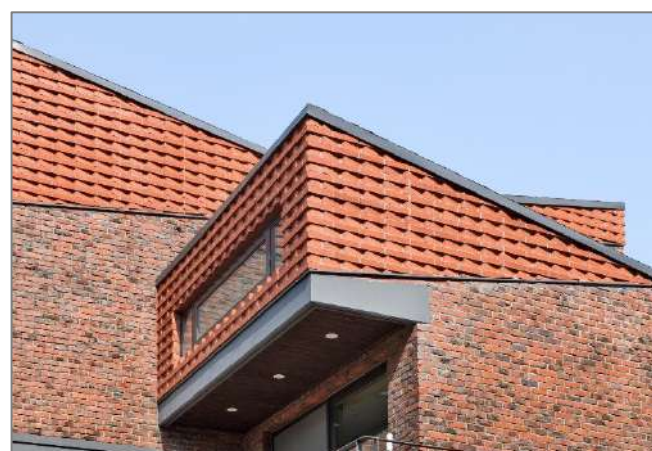
Figure 6: Older brick homes are easy to renovate - by using angled bricks this homeowner extended up a floor and added a contemporary twist.
