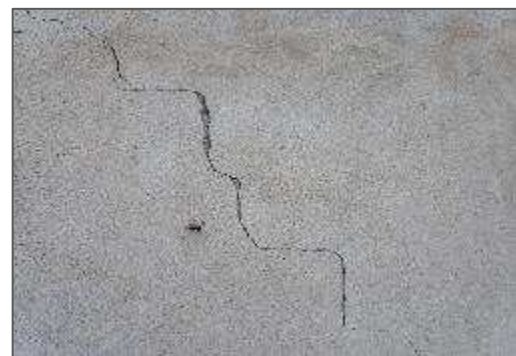
Non-structural Crack
