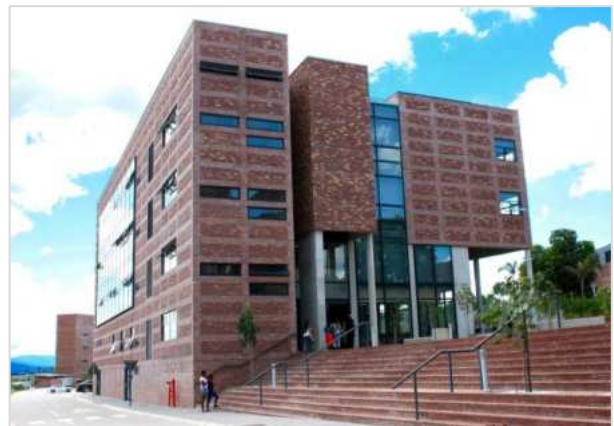
Figure 1: The University of Mpumalanga. Dense clay brick masonry resists the transmission of airborne sound waves. Due to these natural acoustic properties, pupils and teachers are not subjected to excessive noise transmitted from adjoining buildings or classrooms. Photo courtesy of Federale Stene.
