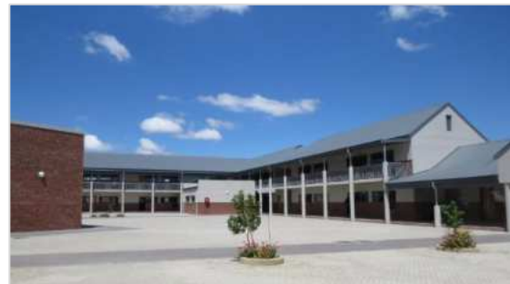
Figure 5: Zweletemba High School in the Western Cape makes extensive use of face brick. This provides an aesthetic, low maintenance finish as well as built in noise and heat insulation. Photo courtesy of Worcester Brick.
